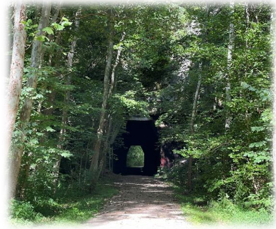
Figure 1: Long abandoned train tunnel
